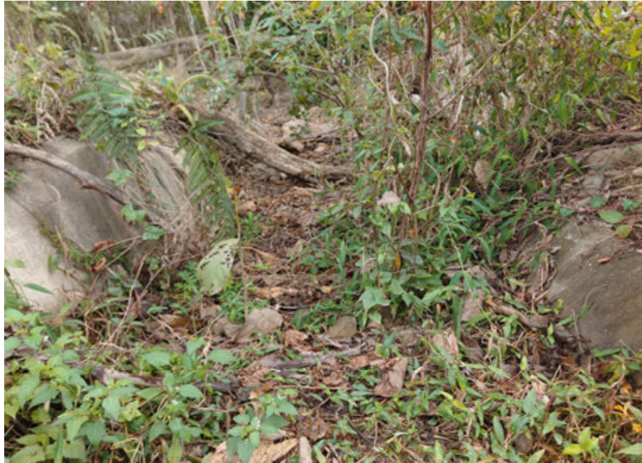
A5 - Existing Drainage Channel
